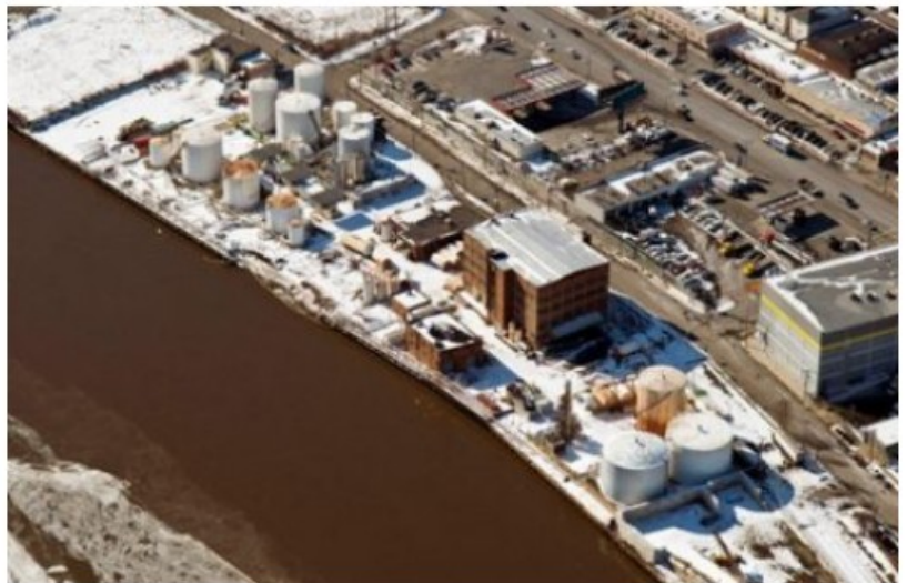
Industrial facility located at 126 Passaic Street in Newark, N.J.
